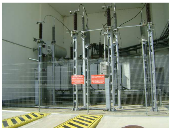
Step-up transformer CoGen
