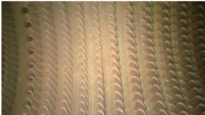
Lower HP casing – center down
